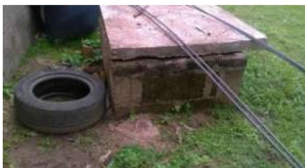
Plate 9: Septic tank with the upper closure slab not properly aligned nor sealed, with openings enough for mosquitoes to hide and rest inside tank-urban.
